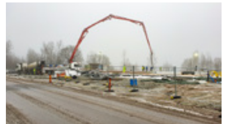
Betongplattan gjuts i decemberdimman.
